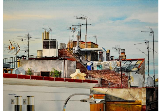
Rooftops of Barcelona by Bob Cook
